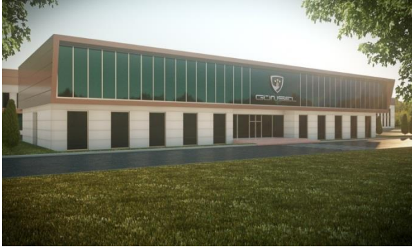
Fig. 1: NEU car factory management building (NEU DESIGN in 2018)
